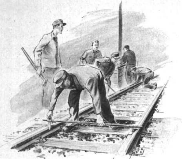
Fig. 3 Measuring the Gauge with a Track Gauge
