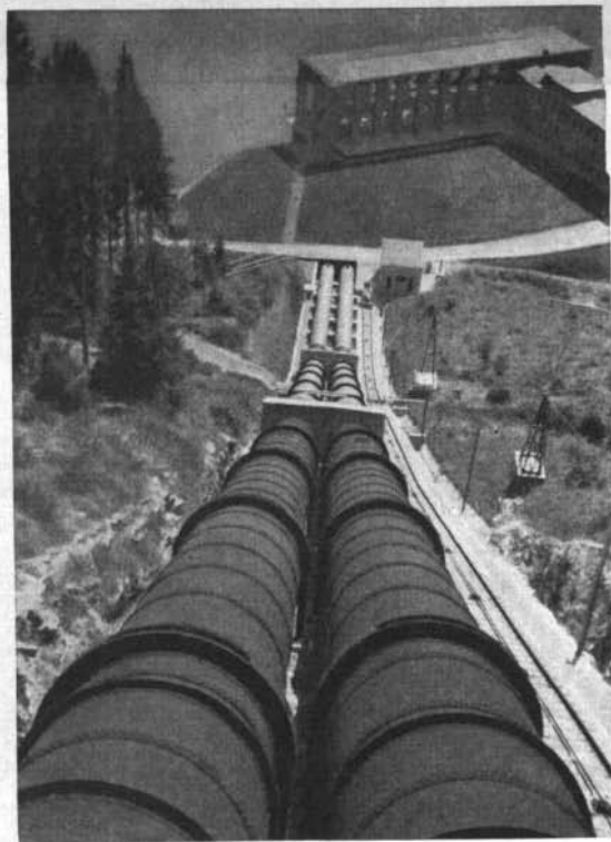
Fig. 73 The Penstocks and Turbine House of a Mountain Hydro-Electric Power Station
